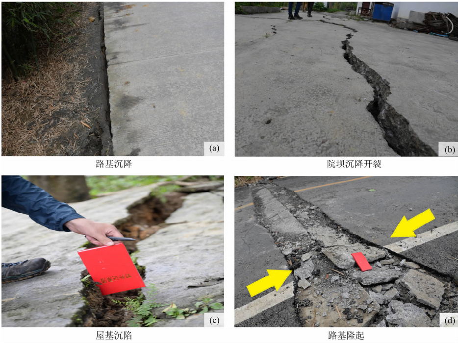
图 6 路基、屋基等变形及破坏特征 Fig. 6 Deformation and failure characteristics of road and building foundation
