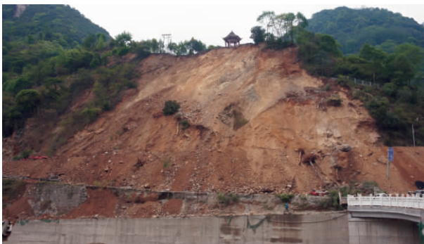
图 5 宝兴县城烈士陵园滑坡毁坏城区道路 Fig. 5 Landslide in martyr cemetery of Baoxing county , destroying urban road
