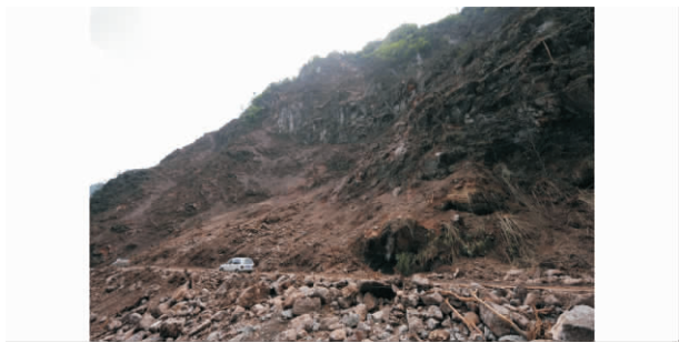
图 2 宝盛乡金鸡峡崩塌落石危害公路 Fig. 2 Rockfalls threatening highway in Jinji gorge ,Baosheng
