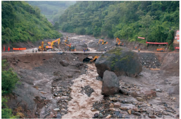
图 6 由于涵洞被堵沟道下游公路桥拦截了大部分泥石流物质 Fig.6 Most of debris-flow sediment intercepted by the road bridge across the downstream channel
