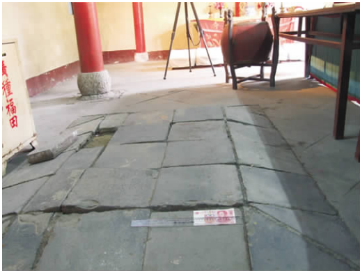
图 2 “活地”尺寸测量 Fig. 2 Measurement of the “growing” terra’s size
