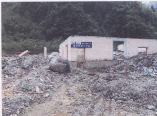
图 3 泥石流冲毁、淤埋房屋 Fig. 3 Buildings buried by debris flow
