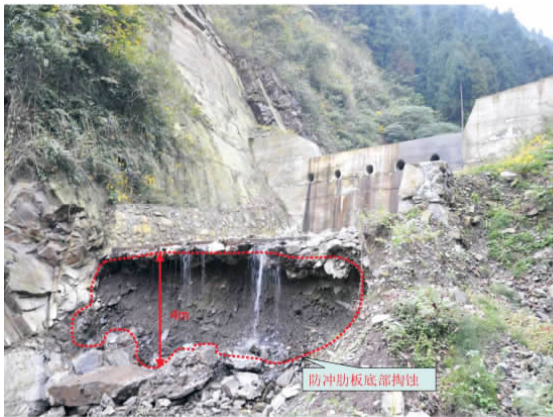
图4 3#坝防冲肋板底部被掏蚀 Fig. 4 Basement of the third dam being erosion
