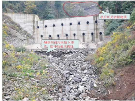
图5 4#坝坝址处以地下渗流排泄水流 Fig. 5 Groundwater seepage beneath the forth dam
